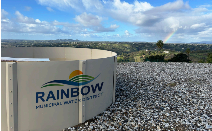
The Pala Mesa Heli-Hydrant was built to assist with fighting local wildfires.
