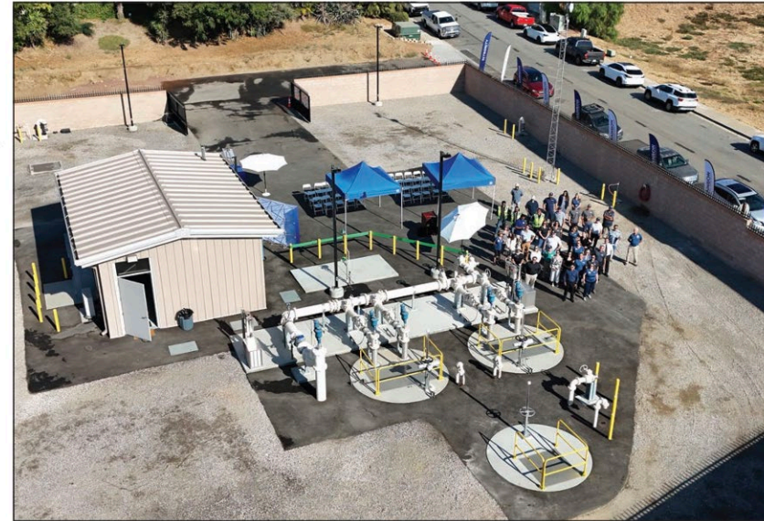
Rainbow Water celebrates the opening of Thoroughbred Lift Station with community and project partners in September 2024.
