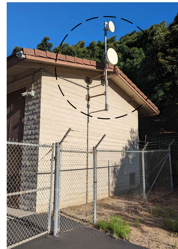
RANCHO AMIGOS PS EXTERIOR POLE MOUNT ANTENNA DETAIL NO SCALE B 10
