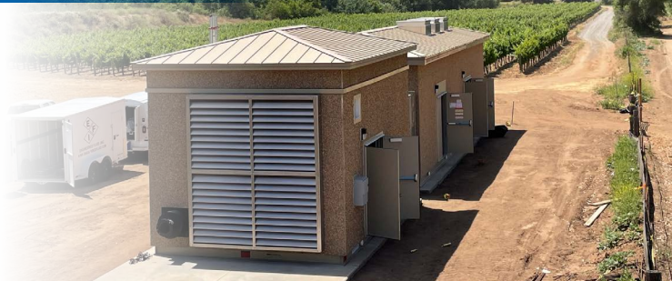
The Rancho Amigos pump station was one of three pump stations recently commissioned to make detachment possible.
