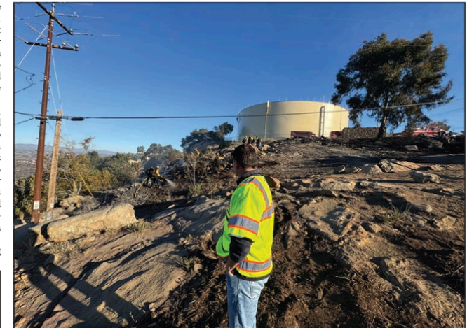
Rainbow Water General Manager Jake Wiley assesses the Lilac fire damage around Hutton Tank in Bonsall.
