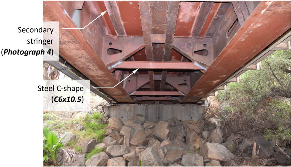
Photograph 2 – Underside of the bridge
